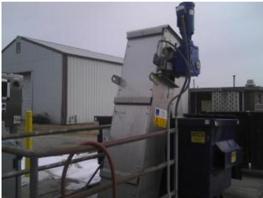
The facility is equipped with a bar screen. Operation of the bar screen is controlled by a depth sensor in front of the screen, and is powered by 1 hp motor. No changes are recommended for this system.
