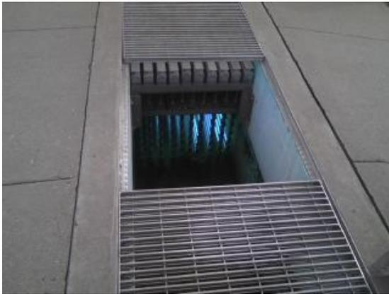
The facility includes two UV disinfection units. Each unit has two racks, each containing 8 high intensity bulbs. The units are on constantly, and there is no means to alter the dosage of the bulbs. They clean the bulbs twice a year, and they get approximately 12,500 hours out of the bulbs. No changes are recommended for this process.
