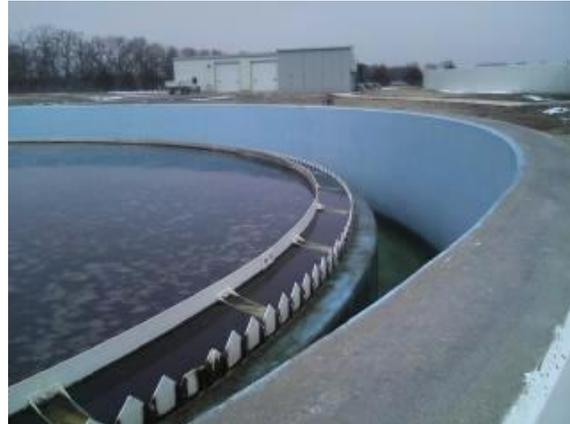
The facility includes two final clarifiers. Each is powered by a 1 hp motor to operate the sweep arms. Each clarifier includes a scum pump which collects scum from the surface of the clarifier and pumps it back to the bottom of the clarifier for additional treatment. No change recommended for this system.
